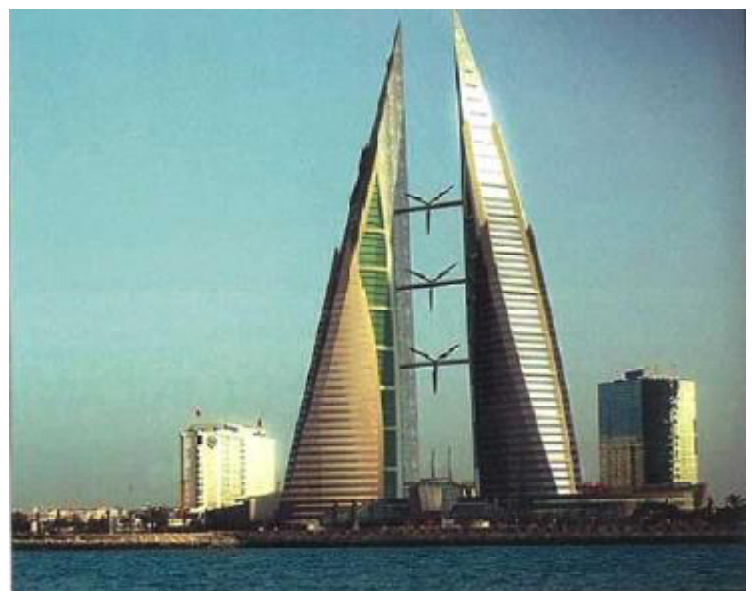
Not expected to be economic: An artist's impression of Nakem's World Trade Centre, now under construction, complete with its complement of 675 kW of on-site wind power generation
